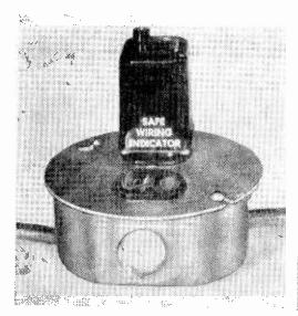
Completed indicator unit shown plugged into AC outlet. Neon bulbs are at top of case.
